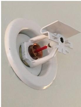
is located in every room of HPP apartments. In buildings with fire sprinkler systems, over 99% of fires are controlled by sprinklers alone. It is extremely sensitive and will release **500 gallons of water a minute** until the system is turned off manually! The last
