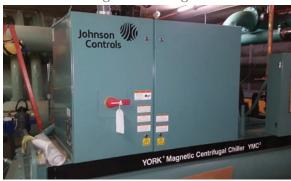
The closed loop chiller system runs 24x7x365 and is estimated to account for about 30% of all electricity consumed by the common elements in our building. The new chiller should run about 30% more efficient and will have a significant impact in reducing our monthly electric bill.
