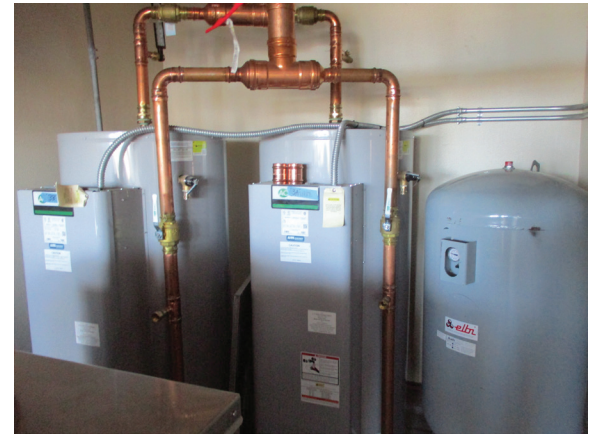
The new heat pumps.
